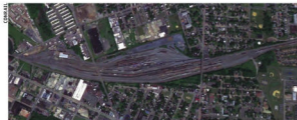
Now operating as a flat yard, the 1.5-mile-long Pavonia facility features 31 classification tracks, nine receiving tracks and eight support tracks.
