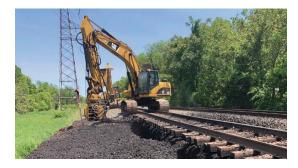
Drainage is one of the most important aspects of track infrastructure. It's important to maintain adequate drainage with proper track ballast to ensure proper cross level, surface and alignment of track. This allows the track to support the loads imposed by rolling equipment.
